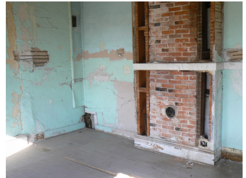
Unfinished interior wall
