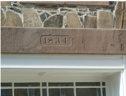
Lintel showing 1834 date
