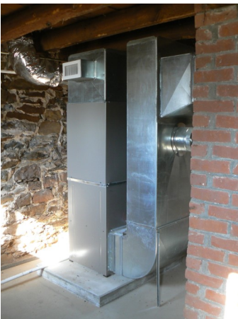
New heating system ducts
