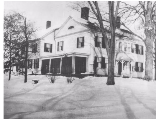
Filley house on Brown Street Courtesy of Caroline Archer
