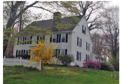
Sanford House, Maple Avenue, 1780 WHS Archives photo
