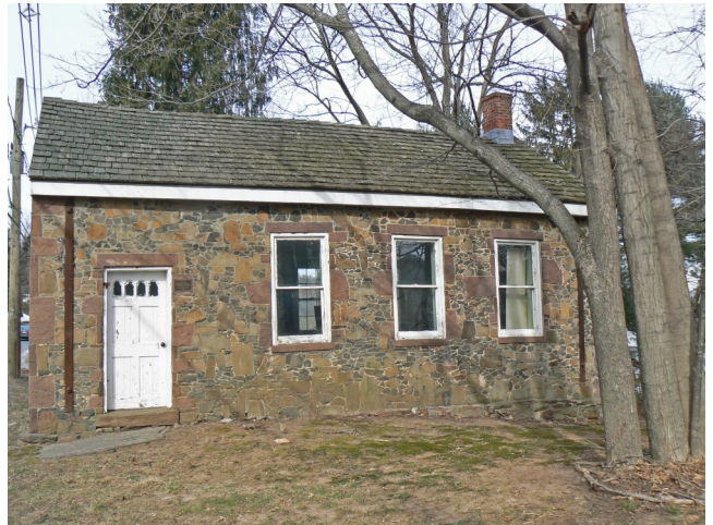
Southwest District School 430 Simsbury Road R. Pierce photo
