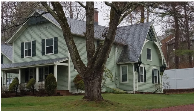
The Gothic revival details at the gable end, right, reveal this house’s origin as the Tariffville Baptist meeting house. —R. Pierce photo
