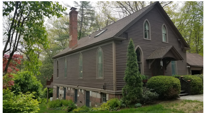
462A Tunxis Avenue, Bloomfield: Notice the unique stone-work of the foundation. —R. Pierce photo
