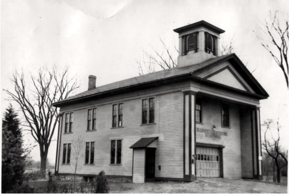
The Academy, rebuilt as a firehouse WHS archives photo
