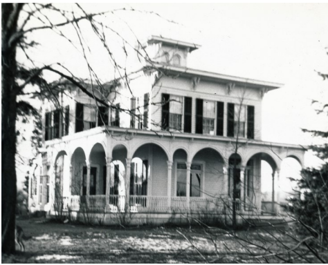
Amasa Jerome House South side of Park Avenue 1939 photo, WHS archives
